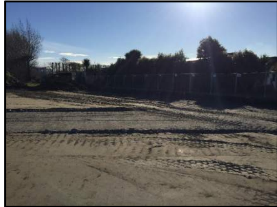
Photo 6: View over Lots 34 to 36. Photo facing northwest.
