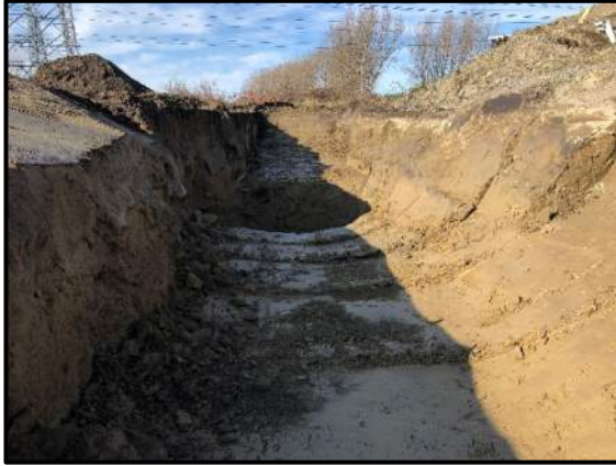
Photo 19: Rubbish trench excavation. Photo facing southeast.
