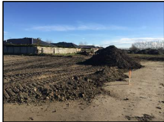
Photo 8: Topsoil being placed on Lot 103. Photo facing west.
