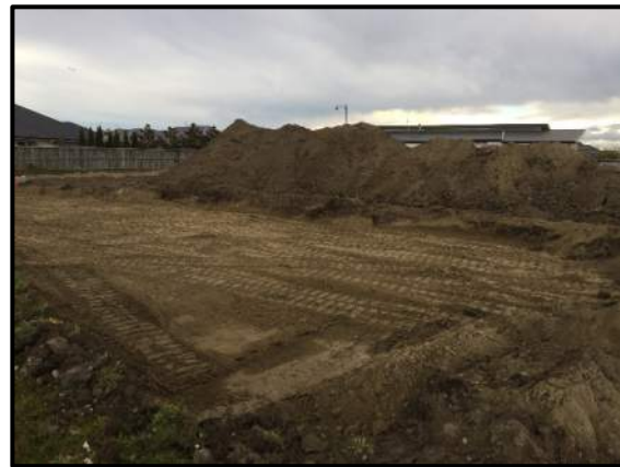
Photo 10: Lot 109 with topsoil stockpiled adjacent to the excavation. Photo facing southwest.
