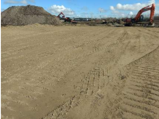
Photo 27: View Lots 73 to 78. Photo facing southwest.
