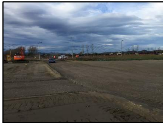
Photo 2: Road 501 had been backfilled with granular fill. Photo facing south.
