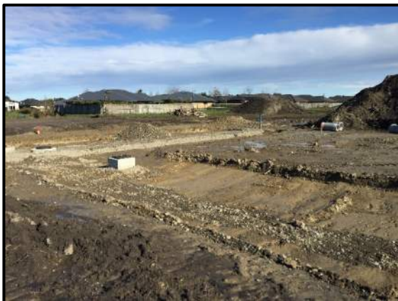
Photo 15: View of the road 501 and adjacent. Photo facing southwest.
