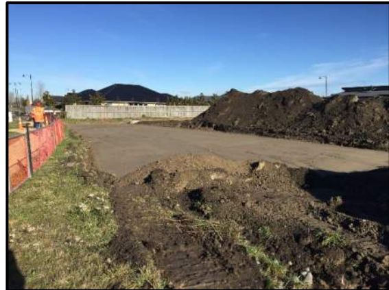
Photo 12: Lot 109 following placement of engineered fill. Photo facing southwest.
