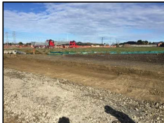
Photo 16: View of the road 501 and adjacent. Photo facing east.
