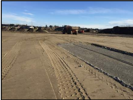
Photo 5: View over Lots 25 to 32 prior to topsoil placement. Photo facing southwest.
