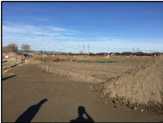
Photo 7: Topsoil placed on Lot 104. Photo facing south.
