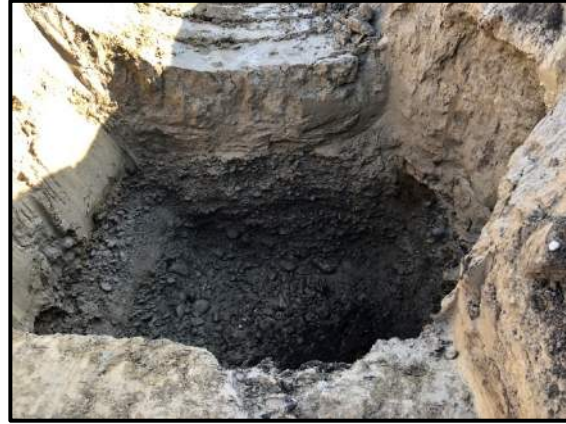
Photo 20: Deepened excavation to gravel layer approximately 2.5 m bgl.
