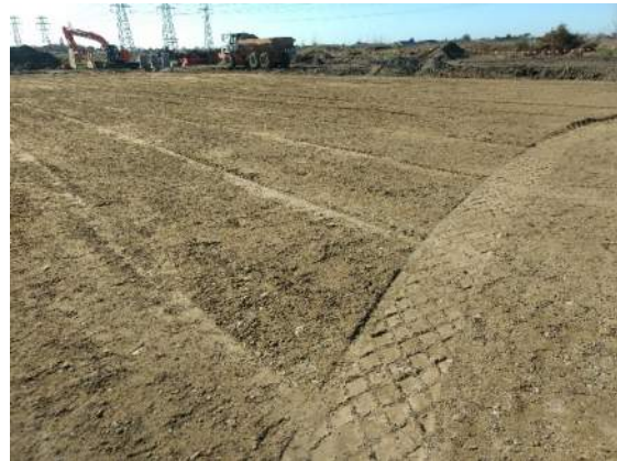
Photo 24: View of Lots 79 to 84. Photo facing northeast.
