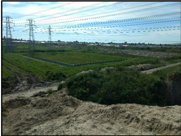
Photo 3: Row of electrical tower pylons with adjacent stormwater retention basins observed. Silt and fill stockpiles observed in the foreground.
