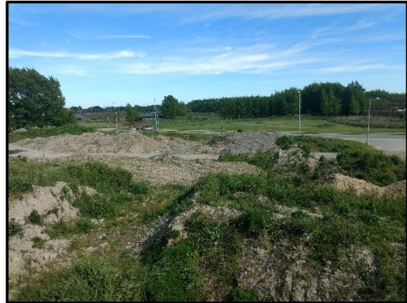
Photo 4: Silt, fill and unknown material stockpiles observed in section 1C of the proposed stage 1 development.
