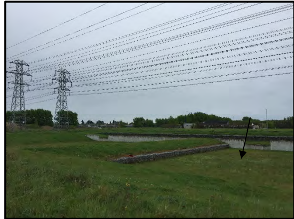
Photo 2: Electrical pylons observed to intersect the subdivision development. Existing storm water retention basins adjacent to the pylons (black arrow).
