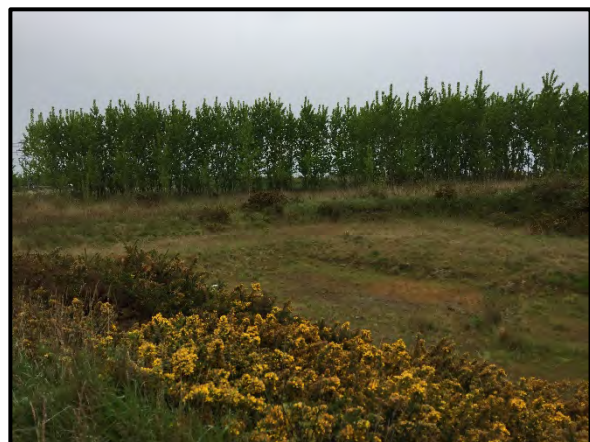
Photo 6: Stormwater retention basin observed in Stage 5C approximately 2.5 to 3 m below adjacent ground level.
